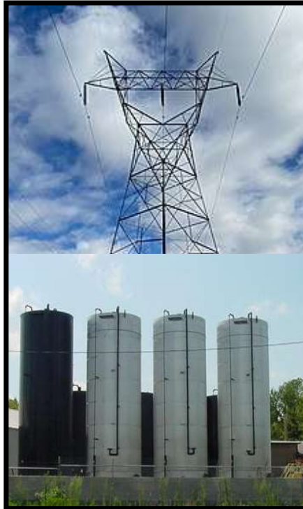
Electrification & demand management
