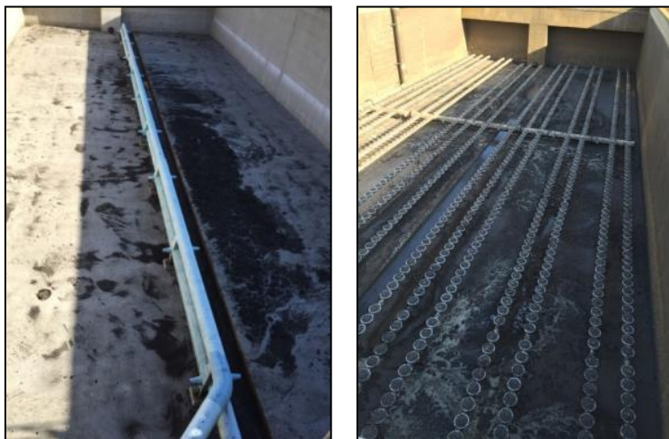
Figure 1. Schematic of high velocity jet aeration pushed through one pipe (left) vs. low pressure fine air bubble diffuser aeration through many discharge points (right)
