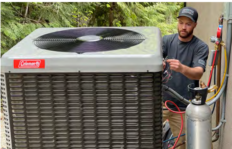
A technician installs a heat pump. Source: Phyxter .
