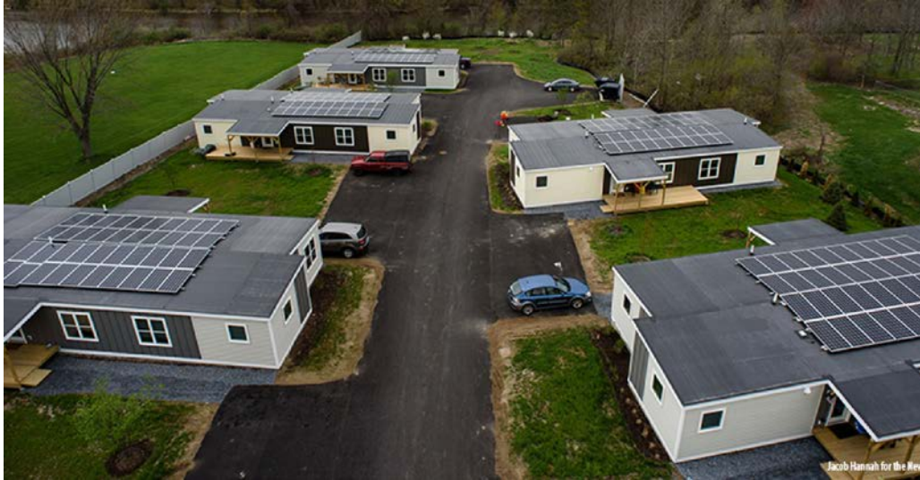
Figure 5. Zero-energy modular homes on McKnight Lane in Waltham, VT. Source: VHCB 2020b.
