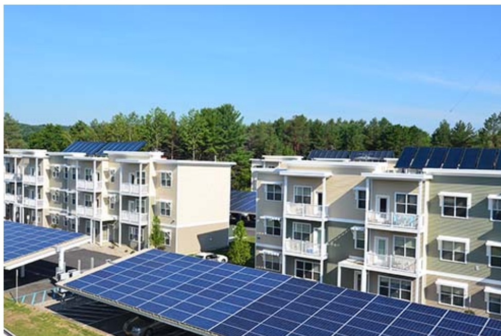
Figure 4. NetZero Village, New York Capital Region (Goodell 2019). This is a low-rise project.
